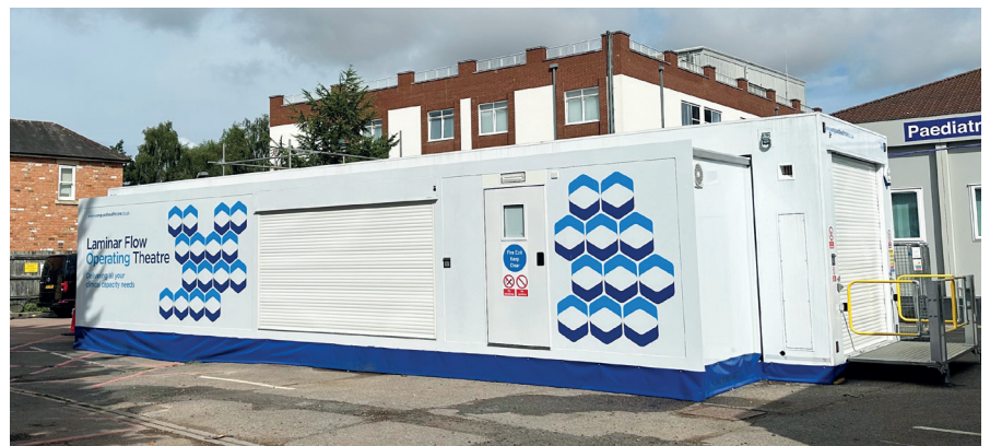
The outside of the Vanguard laminar flow theatre, in position at Warwick hospital.
